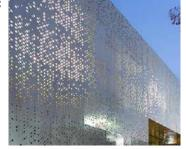
EXTERIOR SHADING SYSTEM (ES1) Material: Perforated aluminum panels Colour: White Pattern: Variable Location: Exterior cladding on Station
