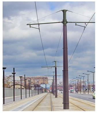
Figure 4-38: Overhead catenary system (OCS) poles
