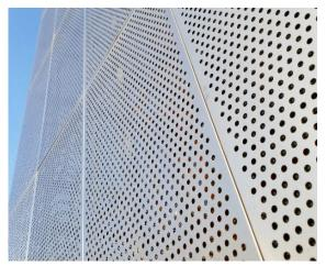
Figure B-2: Perforated Metal Panel
