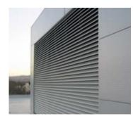
LOUVERS (LV1) Material: Aluminum slats Colour: To match building facade Location: Exterior stations, EEB's, Ancillary Buildings
