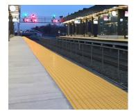
TACTILE FLOORING (TWSI) Material: Integral attention and guidance indicators Colour: Yellow Finish: Anti-slip Location: Platform edges; top of stair/ramps; wayfinding path
