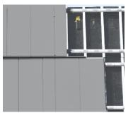
OPAQUE CLADDING (EW1C) Material: Precast and cast in place concrete Colour: Light grey Location: Exterior cladding on Ancillary buildings, EEB's
