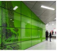
FEATURE WALLS (WF5B - ALT.) Material: Back painted glass, low iron Colour: Variable Pattern: Variable Location: Vertical circulation, platform
