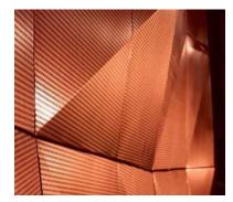
FEATURE CEILING (CF4 - ALT.) Material: Solid and perforated aluminum panels Colour: Variable Pattern: Variable Location: Ceiling(s) at vertical circulation
