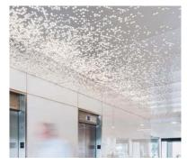
FEATURE CEILING (CF4) Material: Perforated acoustic metal panels Colour: Variable Pattern: Variable Location: Ceiling(s) at vertical circulation
