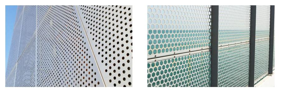
Figure 4-37: Stainless steel perforated sheet for wall screening
