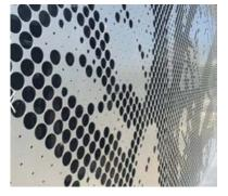
FEATURE WALLS (WF5A) Material: Perforated aluminum panels Colour: Variable Pattern: Variable Finish: Smooth Location: Vertical circulation, platform
