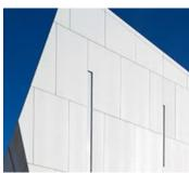
OPAQUE CLADDING (EW1A) Material: High performance porcelain/ceramic panels Colour: Light grey Finish: Matte Location: Exterior cladding stations
